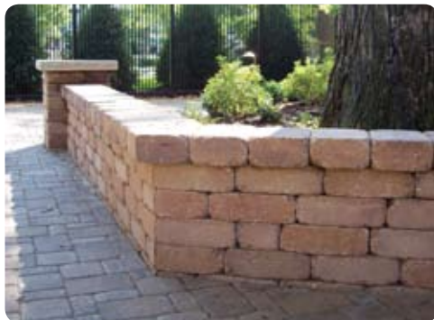
LedgeStone Retaining Wall
