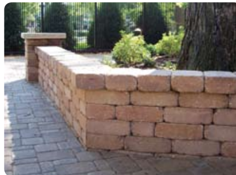
LedgeStone Retaining Wall
