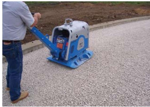
Figure 5. A 13,500 lbf (60 kN) plate compactor includes a device that indicates when no further compaction is needed on the area being compacted. This can reduce compaction time and increase assurance that the PICP open-graded base is compacted.
