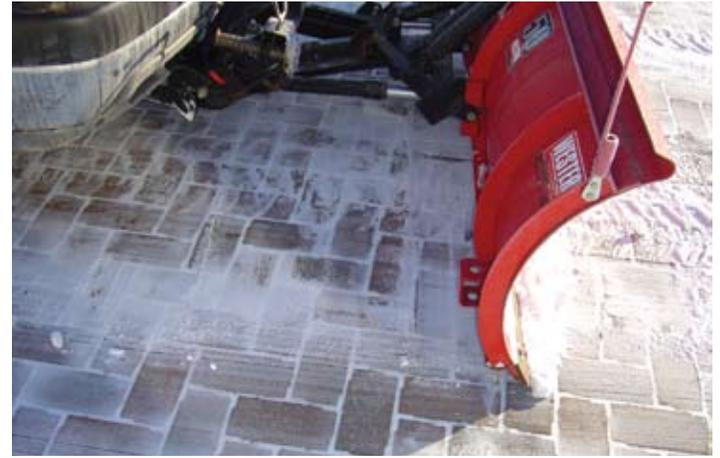
Figure 8. PICP surface openings promote faster snow melting thereby reducing hazardous ice in winter.
