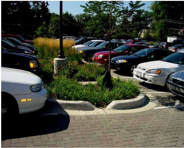
Figure 2. PICP is combined with bioretention to treat runoff from this college campus parking lot in Elmhurst, Illinois. Photo courtesy of ICPI.
