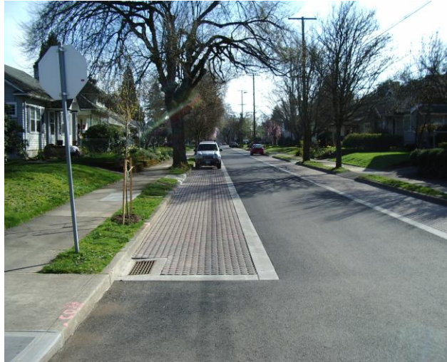
Figure 3. A residential street in Portland, Oregon uses PICP to reduce combined sewer overflows. Photo courtesy of ICPI.
