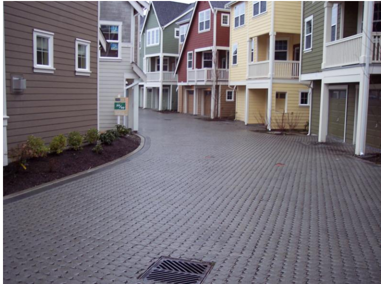
Figure 1. PICP in Seattle's High Point neighborhood significantly reduce the total amount of impervious surface and runoff. Photo courtesy of ICPI.
