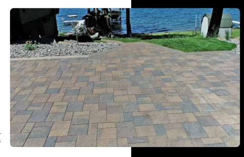
A permeable installation using Select Series pavers ultimately protects waterways while reducing the amount of runoff from impermeable surfaces on a property. Where stormwater falls on a permeable paver system, it percolates back into the subsoil through joints in the paver surface, relying on nature's filtering system to prevent runoff and heat island effects and protect aquatic ecosystems, while supporting pedestrian or vehicle traffic.
