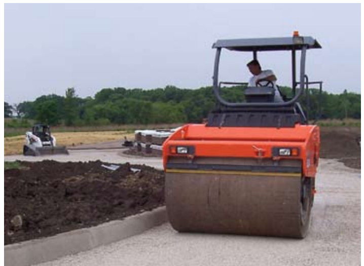
ICPI is evaluating test methods for measuring density and stiffness of PICP open-graded bases using the classic vibratory roller shown here and large plate compactors.
