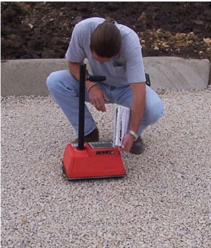
Figure 1. A common site on pavement construction: a technician reads a nuclear density gauge on and PICP project.
