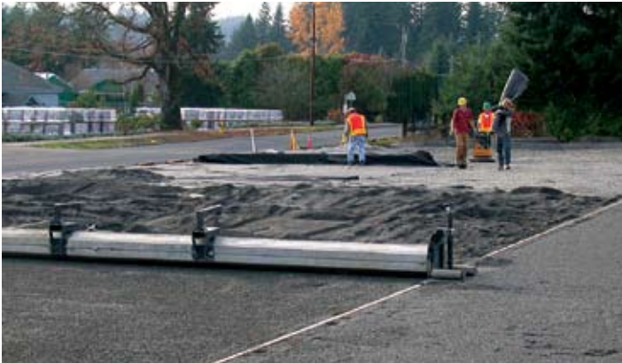
Figure 7. Mechanical screeding of the bedding material speeds construction on larger projects.
