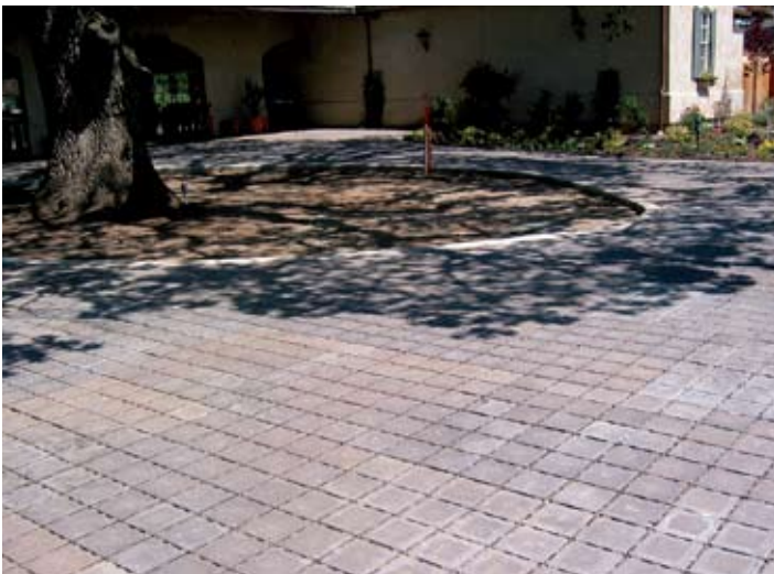
Figure 6. Like all permeable pavements, PICP can extend tree life by sending air and water to the roots. An additional sustainable aspect is paving units can be made with cement substitutes and recycled concrete.
