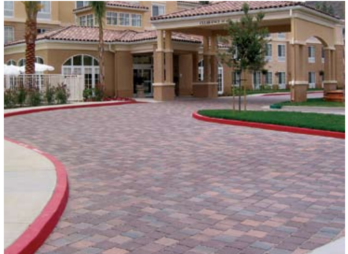
Figure 5. PICP color and texture compliments the architecture of a Hilton Garden Inn in Calabasas, California while communicating the sustainable nature of the site.
