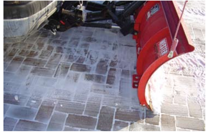
Figure 9. PICP is snow plowed like any other pavement.
