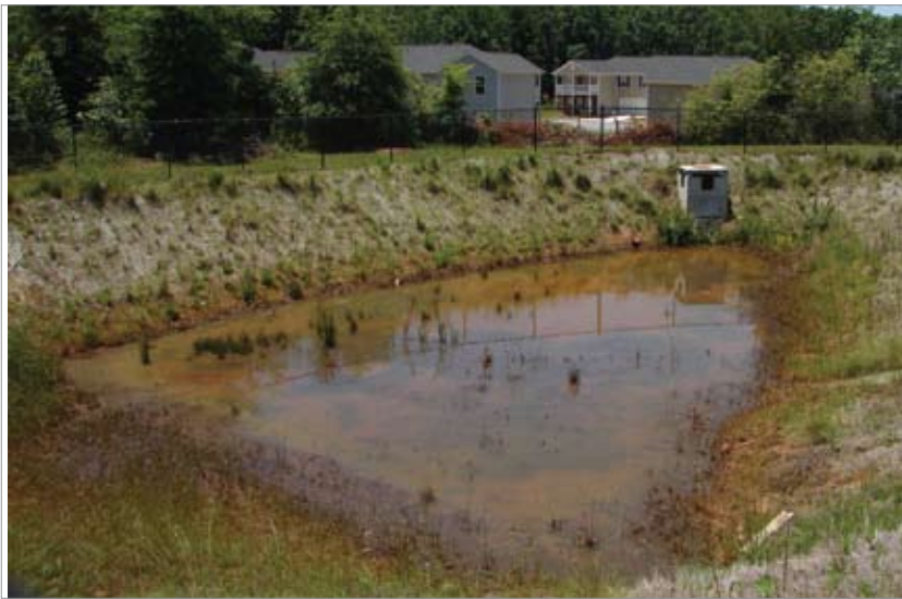
Figure 1. On-site infiltration practices such as permeable pavement are emerging as preferred stormwater management solutions to off-site controls such as detention (shown above) and retention ponds that consume valuable land. PICP can reduce or eliminate these facilities.
