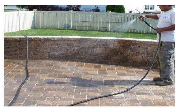
Step 11: Check joints to make sure sand is moist (3/4" - 1")
