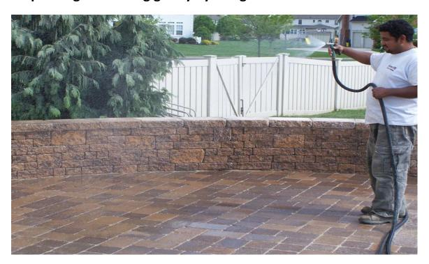
Step 10: Gradually add more moisture 3-4 times. Stop when you see any foam in joints (floating polymers). \*Use a leaf blower to blow any excess water off textured pavers
