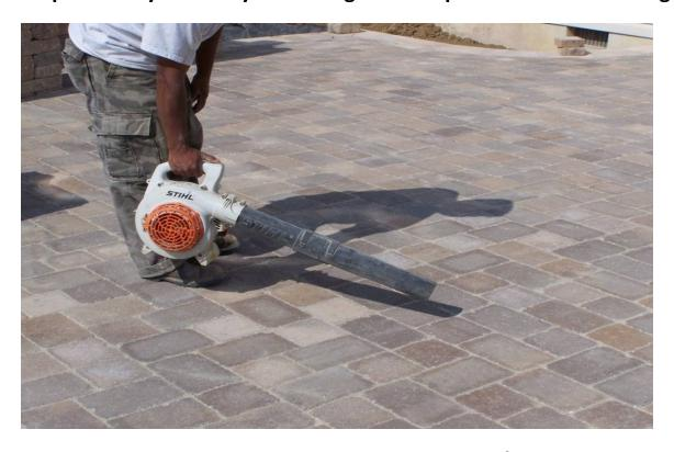
Step 8: Sand should be at bottom of chamfer or 1/8" from top
