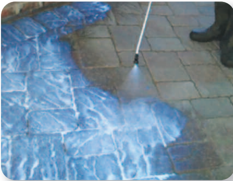
FLOOD COAT & SQUEEGEE Application Method to Be Used with Joint Sand Stabilizing Sealers
