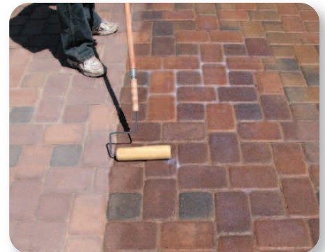
SPRAY & BACK-ROLL Application Method to Be Used with Wet Look Sealers, Special Use and Invisible Penetrating Sealers
