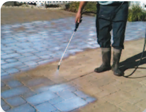
SPRAY & BACK-ROLL Application Method to Be Used with Wet Look Sealers, Special Use and Invisible Penetrating Sealers
