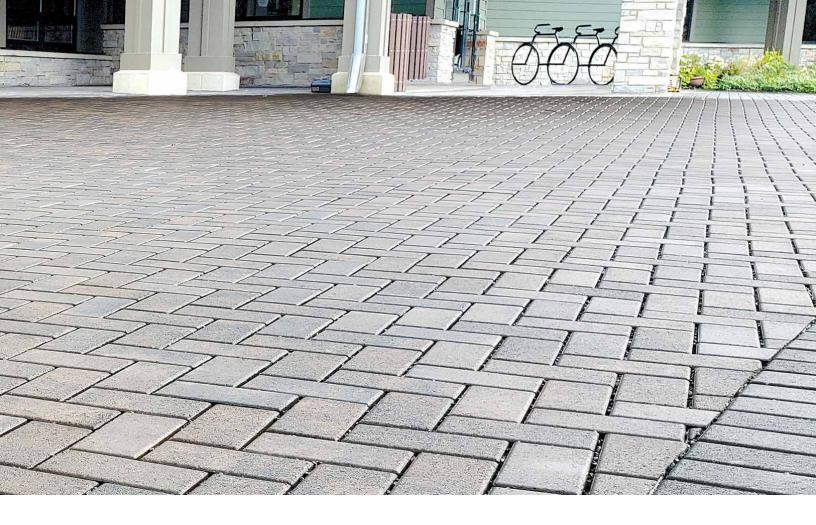
NOTE: PICP systems should not be used on sites where stormwater infiltration could contaminate groundwater. Such sites include fueling and hazardous materials storage stations or high water tables, where soil is not deep enough to adequately filter pollutants.
