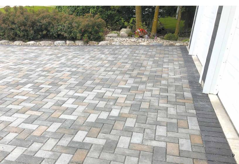
PICP surfaces and adjoining pavement surfaces will require standard structural BMP practices for pavement maintenance regarding sweeping procedures. A vacuum sweeper may be used during dry periods to remove encrusted sediment, leaves, grass clippings, etc. Vacuum and sweeper settings may require adjustments to prevent uptake of aggregate from the paver voids and joints. Water is not used while vacuuming.
