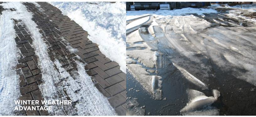
Melting snow drains immediately through permeable pavers, eliminating the risk of re-freeze.
