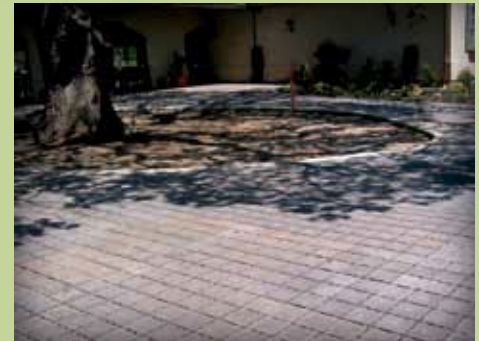
Figure 6. Like all permeable pavements, PICP can extend tree life by sending air and water to the roots. An additional sustainable aspect is paving units can be made with cement substitutes and recycled concrete.
