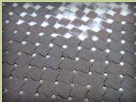
Figure 8. PICP surface openings promote faster snow melting thereby reducing hazardous ice in winter.
