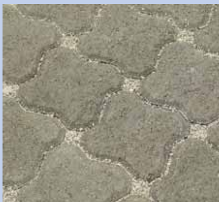
Figure 3. Left to right: After excavation, PICP construction begins with placing and compacting a clear, crushed stone open-graded subbase and base as shown in the first two photos. The next photo shows mechanical installation of the concrete pavers on a screeded bedding layer of small, clear crushed stone. The rightmost photo illustrates small aggregate in the openings and joints that enable high surface infiltration. The pavers and aggregate are compacted to create an interlocking pavement.
