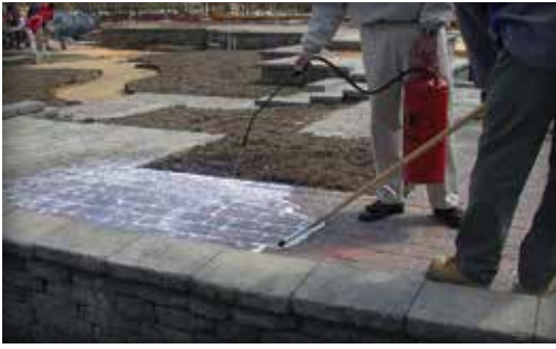
Figure 3. This liquid joint sand stabilizer is applied with a low-pressure sprayer and squeegeed across the surface after allowing some time for soaking into the joints. This helps maintain slip and skid resistance of the paver surface.
