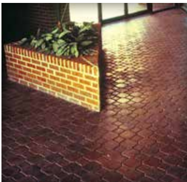
Figure 1. Many sealers enhance the appearance of concrete pavers and protect against staining.
